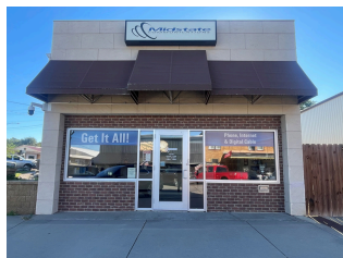
The Chamberlain office before the recent exterior upgrades.
